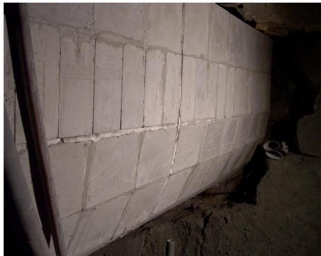
The picture shows a precast bull's nose of D59A
